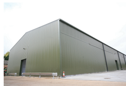
New steel framed building with vented cladding housing 12 stores.
